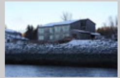
Boardwalk Hotel 12 Unit Waterfront Hotel $795,000
