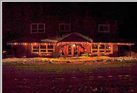
2nd Place C-Ber Building jointly decorated by Central Suites of Seldovia and Yesterday's
