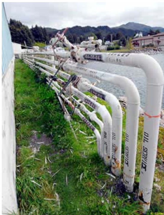
Fuel lines to be replaced from the City Office to Seldovia Fuel & Hardware
