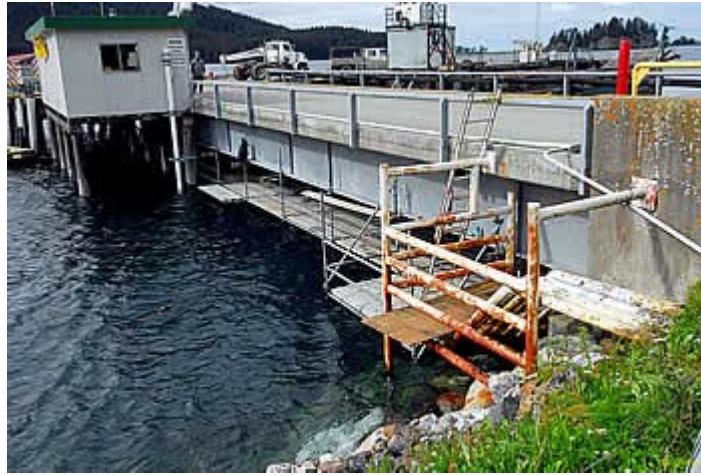
Scaffolding is currently being installed
