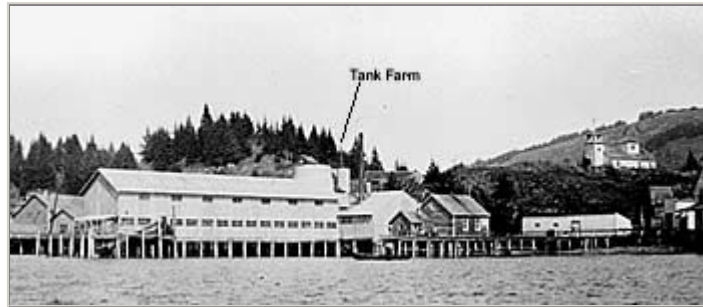
The Tank Farm is visible in this 1933 photo of the Seldovia waterfront. Photo courtesy of the Alaska State Library, Early Prints Collection, #01-2563
